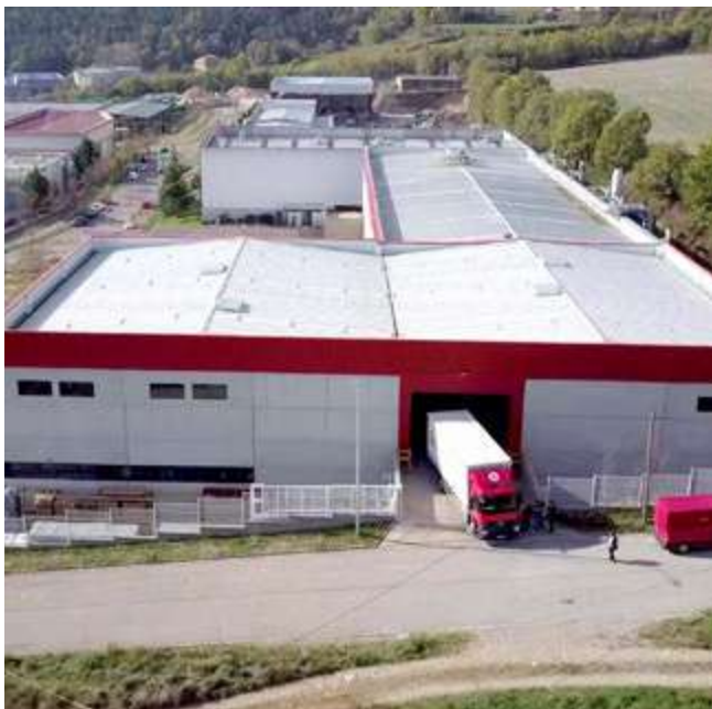
Technical textiles plant. Berga, Barcelona.
