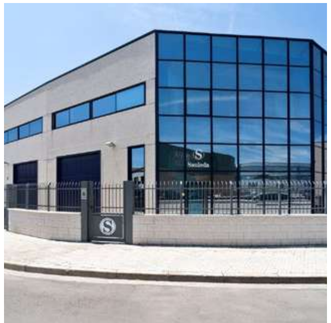
Logistic platform. Malgrat de Mar, Barcelona.
